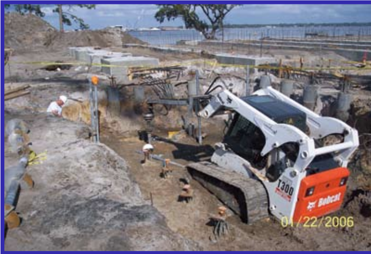
Installation of Drive Rite 26000 Series Helical Piles
