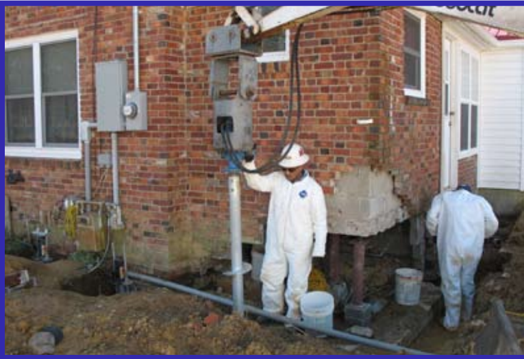
Helical Piles Driven and Terminated at 5,500 ft/lbs. of Torque
