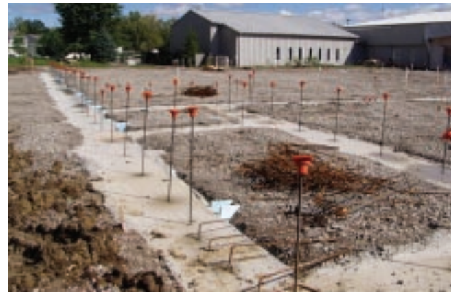
Steel rebar was then placed over the top of the piers in the footer; concrete was poured in the footer trench to ground level.
