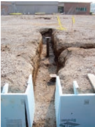
Once the footer crew dug the trench, the piers were cut for the second time. All piers were filled with concrete. Where piers had a final cut at a pipe junction, bolts were installed in the concrete and the bracket was attached to the pier.
