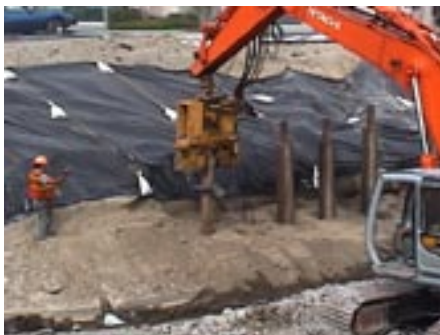
Driving HEATanchors helical soldier pile.
