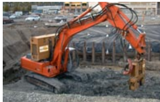
HEATanchors quickly mobilizes into action.
