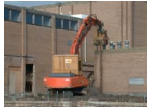
HEATanchors vibration free installation while class is in session.
