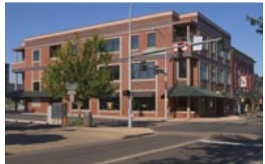
HEATanchors supports the finished Truitt building .
